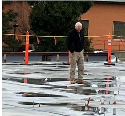
January 19, 2024: Greg Kidder inspects the newly poured slab:
